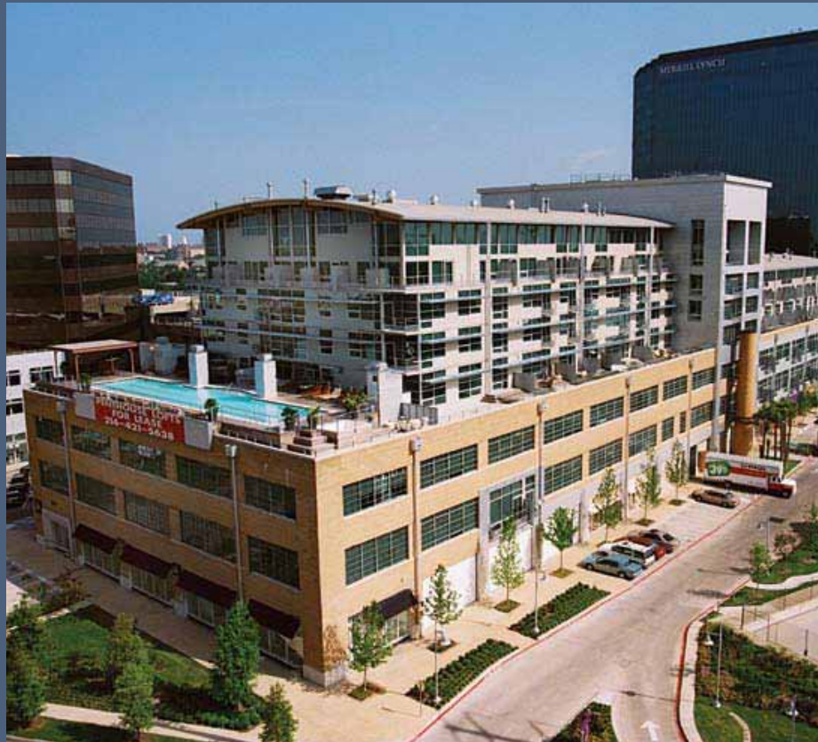
The Lofts at Mockingbird Station - Dallas, Texas This 211-unit urban loft community includes split-level lofts, flats and exclusive penthouse floor plans. As a mix of an existing warehouse renovation and new construction, the property features 178,000 SF of retail and 138,000 SF of office space and is located adjacent to the DART light rail metro transit system.
